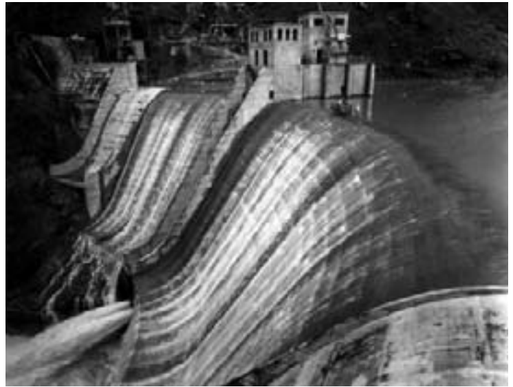
c. 1955. The Anchicaya dam and power station serve the fast-growing city of Cali and were financed by loans from the World Bank totaling $8.03 million.
